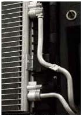
A/C Lines at Condenser
